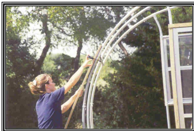
Clamps can be used to hold 1x2 wood strips as the are bent around the end hoops. Remember only the end hoops get the 1x2 strips. If wood is hard to bend, you can kerf the strip. This is simply cutting across the strip about 1/3 through every 1 to 2 inches.
