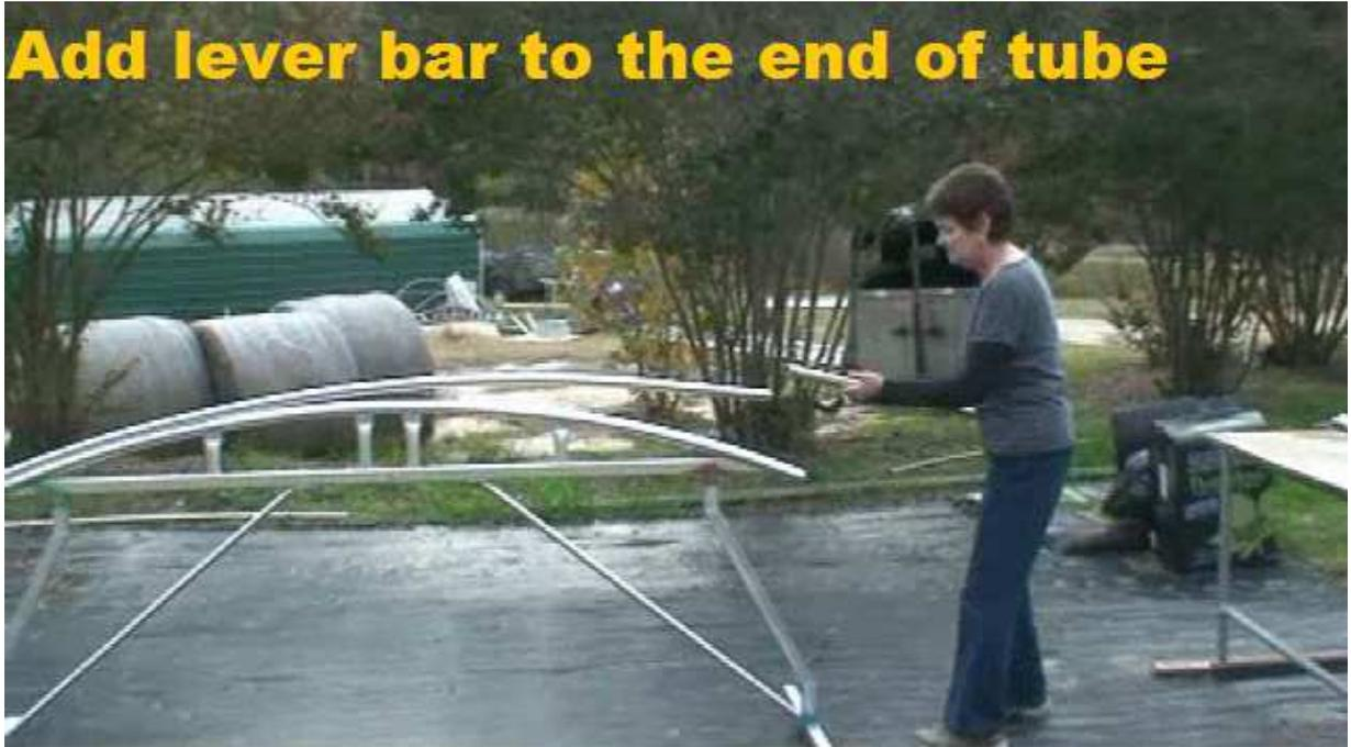
**Pull down until the junction of bar and tube touches the bender**
