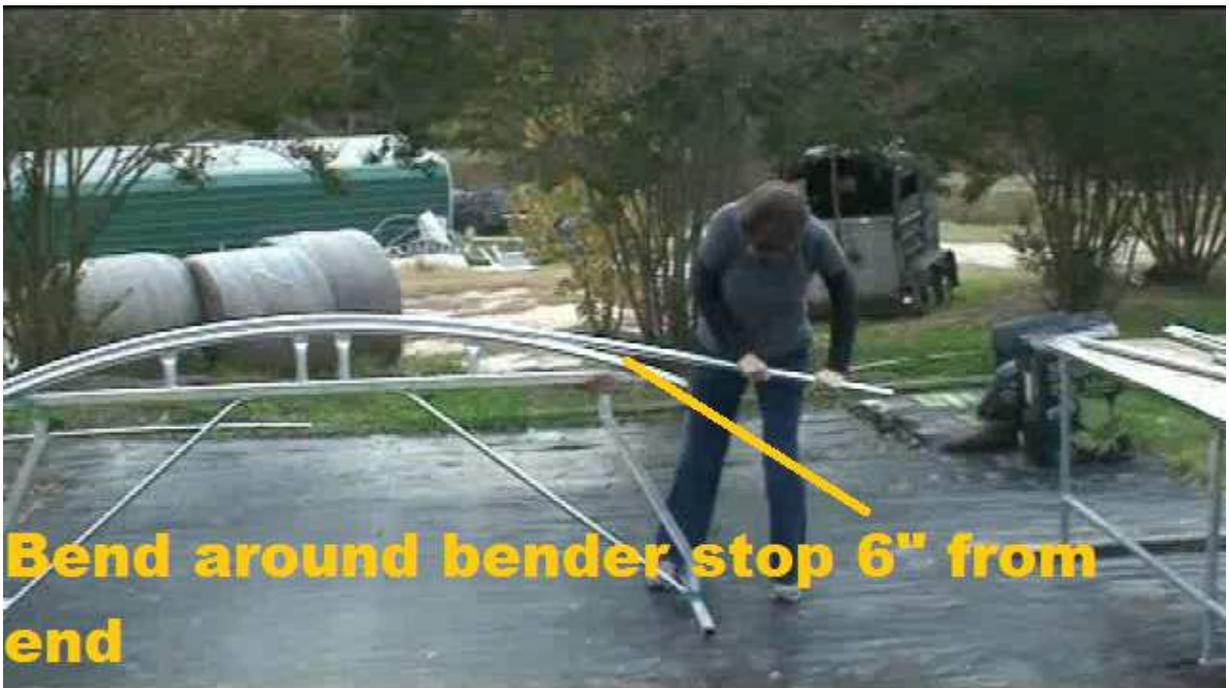
**Push thru strap until end of tube is about 6" to 8" from end**
