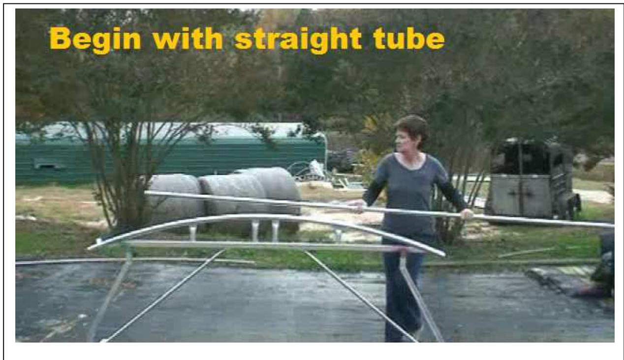
These bending steps are used for building a round 24 ft wide hoop at 11 ½ feet tall in the center, and also used for bending the hoop sections for our 16 ft wide Mono Gothic as well. The 24 ft wide round hoop requires four 10'6" lengths of 1 3/8" O.D. fence top rail tubing either 16 or 17 gage.
